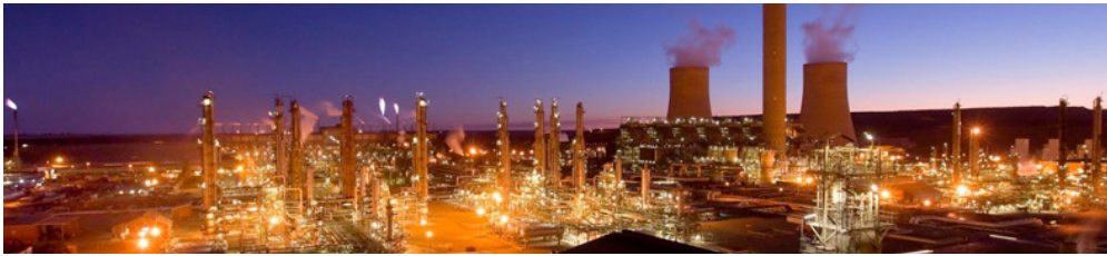
Sasol's Lake Charles Gas-to-Liquid and Ethane Cracker Complex, USA
